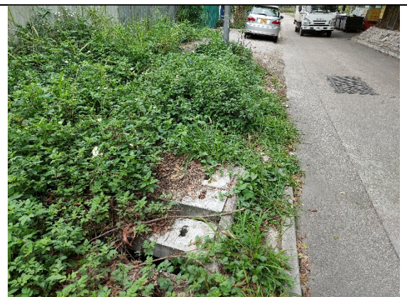
Plate No. 6 – Existing Catchpit 2 which should receive flow from an existing 450U channel and discharge into an existing 525mm diameter drain with respect to the GEOINFO Map
