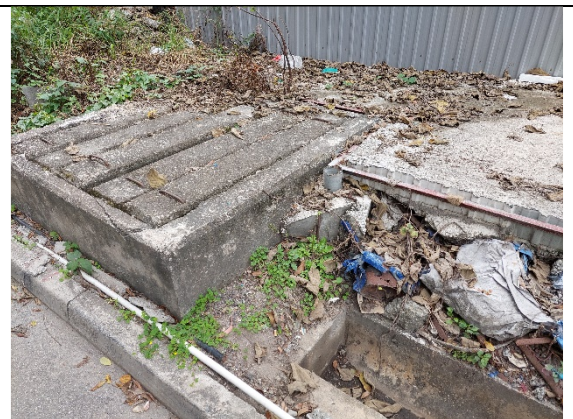
Plate No. 4 – Existing Catchpit 1 and the adjacent existing U channel which is separated from the Existing Catchpit 1 and conveys flow toward Castle Peak Road – Hung Shui Kiu
